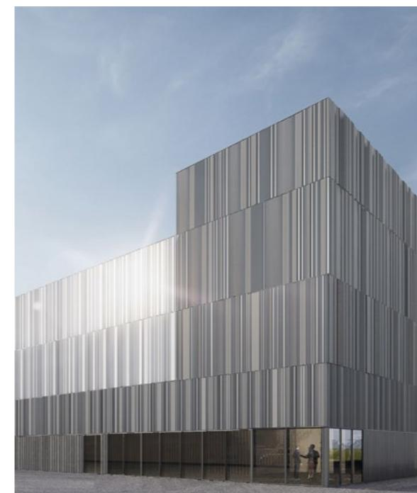
The design of the buildings harmonizes the disparate heights across the site through a layout of horizontal bands intersecting a double-skin steel cladding in metallic gray. The varied cladding profiles create a play of reflections and a vibration of warm tones that blend seamlessly with the office façades.
